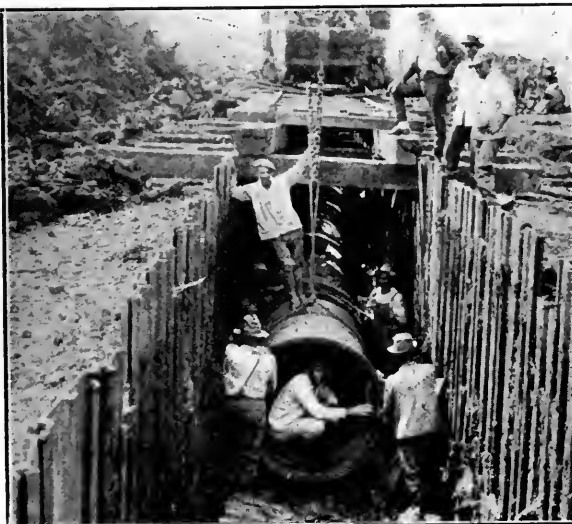
TYPICAL PIPE-LAYING CONDITIONS IN NEW ORLEANS
